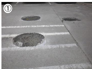
Hole repair test in the rain
