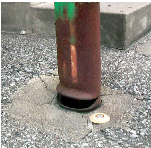
Corrosion of the root portion of the steel street light. Taking advantage of adhesion to the steel, EAGLE8 filling and external neck wrapping repairs .
